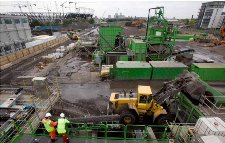
One of the two soil hospitals which formed part of the enabling works, processing tonnes of contaminated soil to be reused on site to create the landforms and remediating the ground for future land uses
