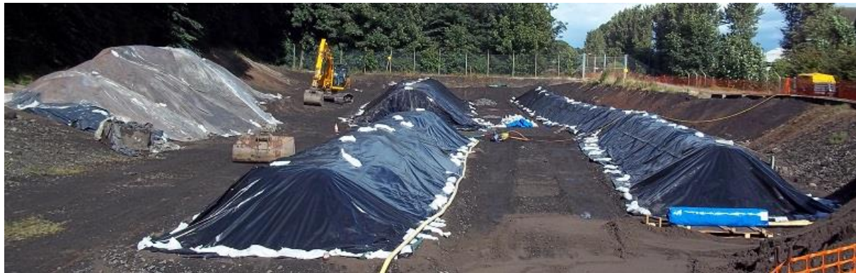
One of the two soil hospitals which formed part of the enabling works, processing tonnes of contaminated soil to be reused on site to create the landforms and remediating the ground for future land uses
